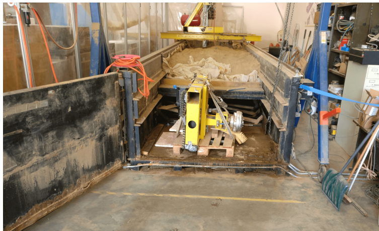
Figure 6.4: Access created for the forklift
