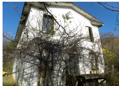
(Above) Evidence of second story floor joists. (Below) South facade of remaining structure.
