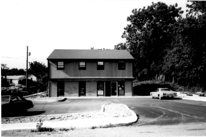
Quick Market/Apartment Structure on Turner Street
