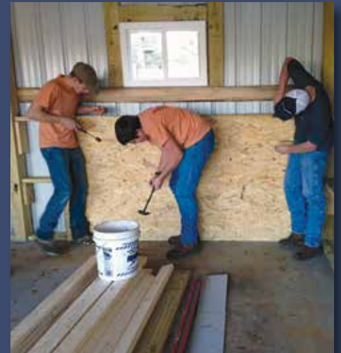
Holston High School students played an important role in finishing the inside of the barn that was built using the grant funds. Once the structure was up, they constructed walls and sides to keep the animals safe.
