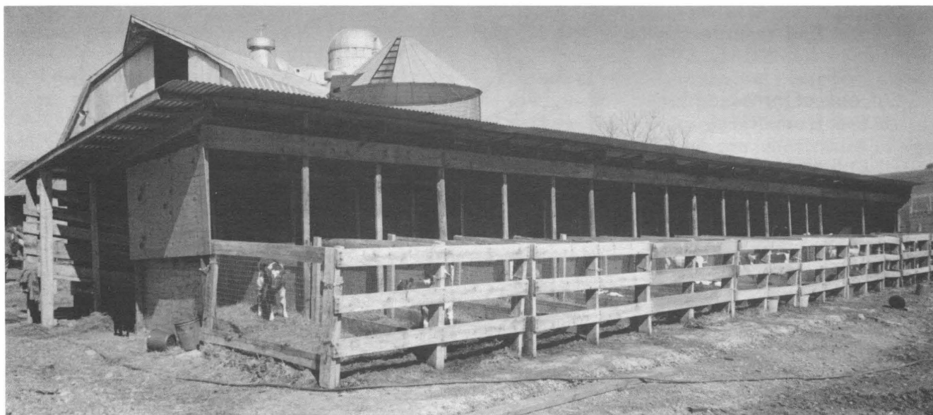
Figure 11. Cold calf-housing systems of this type offer many advantages. Mortality rates are usually very low. They are reasonable in cost and offer efficiency of labor and management.
