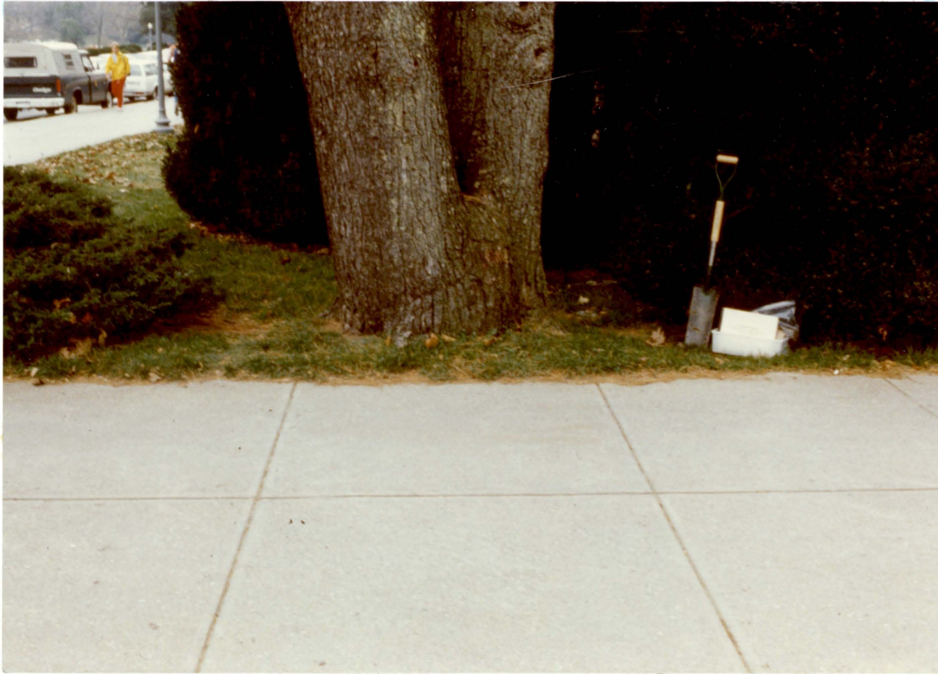
Figure 17: Root disturbance and cover by concrete sidewalk around decline habitat tree (#6) on the Virginia Tech campus.
