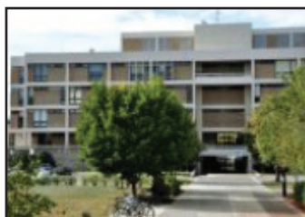
Derring Hall Opened 1969
