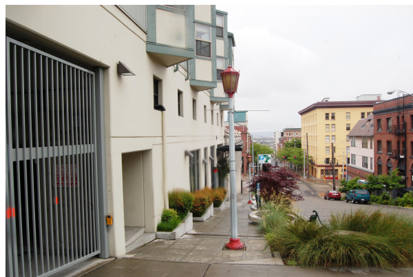
Figure 6.26. Downspout from the building and grated drain connected to the underground cistern.
