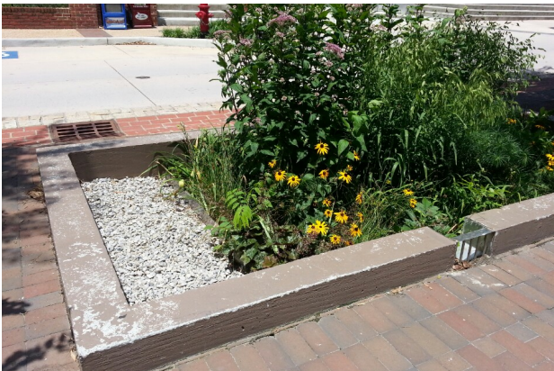
Figure 6.33. Stormwater planter in detail.
