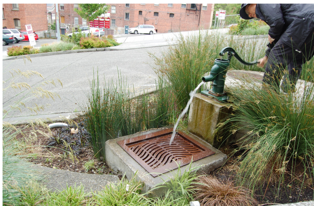
Figure 6.25. Japanese hand pump connected to the underground cistern for irrigation.
