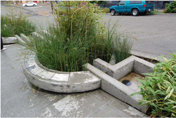
Figure 6.27. Stormwater planters connected with conduit and seating with historical art tiles.
