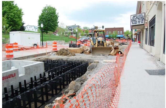
Figure 6.34. Maintaining access to local businesses during construction.
