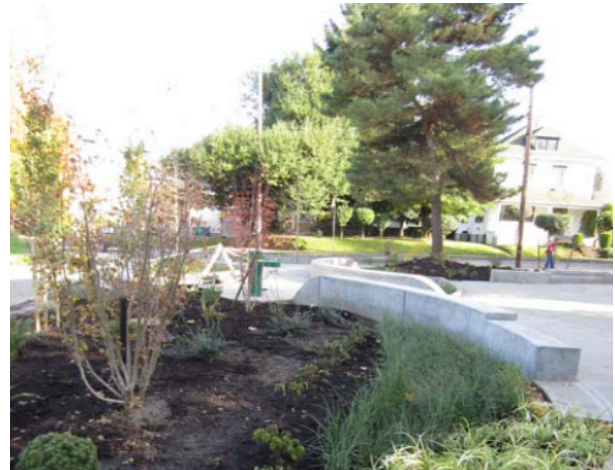
Figure 6.22. Infiltration basin with seat walls and newly paved pathways. Reprinted from Holman Pocket Park and Green Street Bike Boulevard Project (p. 2), by City of Portland. Copyright by City of Portland, OR, courtesy Bureau of Environmental Services. Reprinted with permission.
