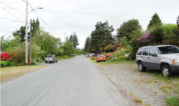
Figure 6.17. Typical residential street before Green Street construction.
