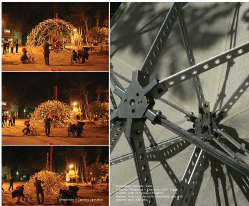
Figure 32: Deployable Geodesic Dome
