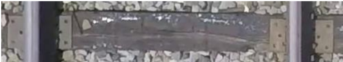
Figure 63. Tie Plate Spike Inspection Image (Altitude: 8 m) – Slight loss in sharpness when compared to the 8 m image, but all tie plate features are still clearly visible
