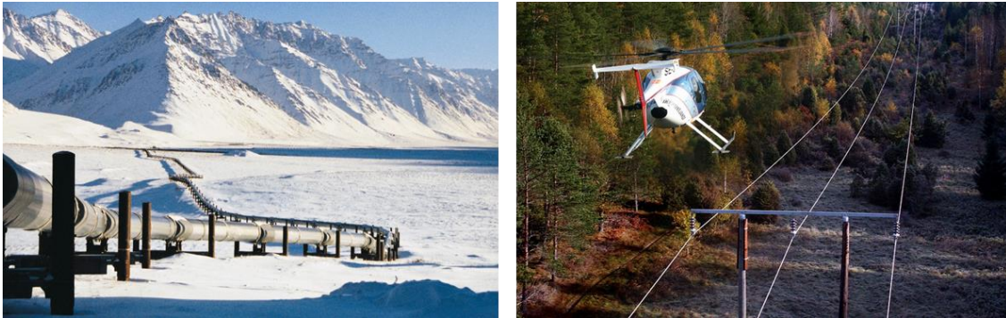
Figure 1. Remote Infrastructure Examples - Example of remote pipeline (left) and power lines (right) presenting inspection and repair challenges
