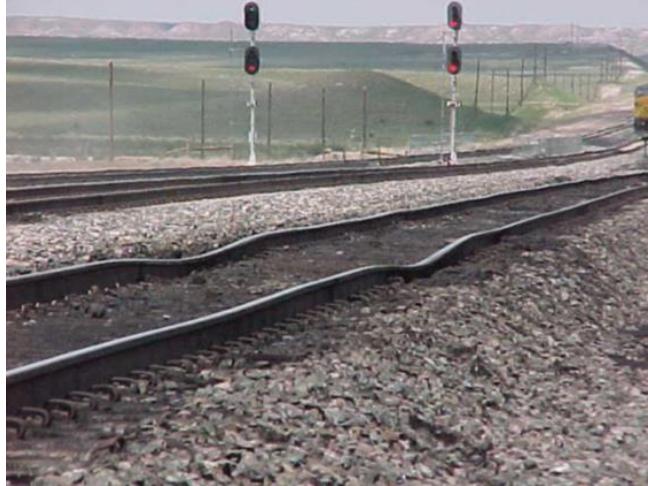
Figure 41. Example of a Rail Kink
