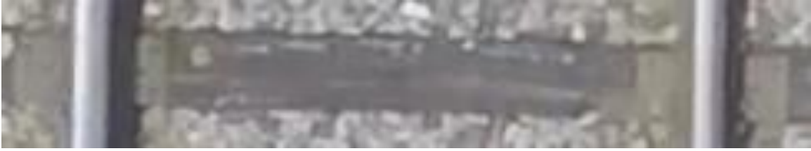
Figure 65. Tie Plate Spike Inspection Image (Altitude: 17 m) – Extensive preprocessing would be mandatory to detect tie plate features, with some tie plate features already becoming invisible
