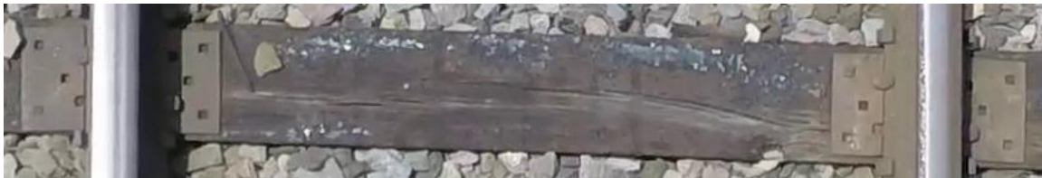
Figure 62. Tie Plate Spike Inspection Image (Altitude: 5 m) – All tie plate features are visible and textures are sharp indicating that GSD is sufficient at 5 m
