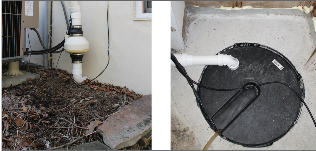
Second radon remediation installation in my house in 2012. On the right, a PVC pipe is installed through the sump pump lid, and on the left, it penetrates the foundation wall and is connected to an exhaust fan named R2D2. Spray foam was injected behind the perimeter drainage angle to close the air gap. The adhesive lines on the wood furring strips are likely left over from when one of the seven previous owners tore down wood paneling installed by an earlier previous owner.
