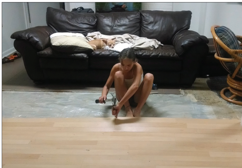
Left, the elder investigative Chihuahua looks on with rapt attention as my daughter removes the rest of the Pergo. Upper right, a tiny leveling-compound ramp used to feather the edge of asbestos-containing floor tile. Lower right, collecting tile and mastic samples for the lab.
