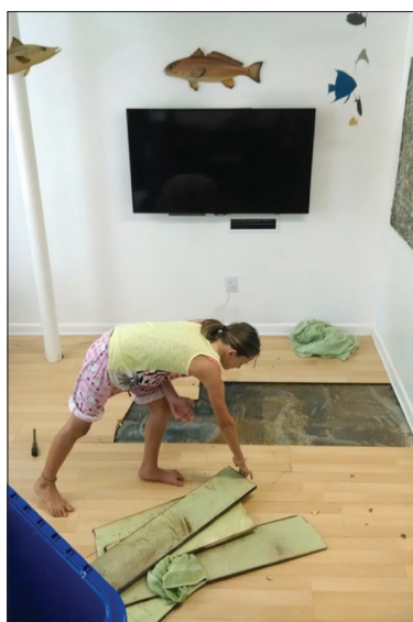
Left , my daughter removing the first of the Pergo boards in the affected area. Gloves (and shoes) are for sissies! Upper right , gross worms on the back of Pergo. Lower right , worms, mud, and God knows what else between the polyethylene sheeting and the floor slab.
