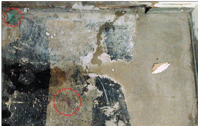
Food coloring experiment to determine the source of the leak.
