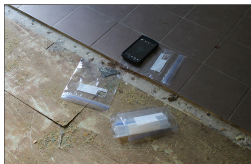
Left, the elder investigative Chihuahua looks on with rapt attention as my daughter removes the rest of the Pergo. Upper right, a tiny leveling-compound ramp used to feather the edge of asbestos-containing floor tile. Lower right, collecting tile and mastic samples for the lab.
