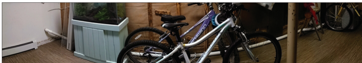
Above, the new sewage pipe runs downward from the kitchen drain (at left), slopes under the ceiling of the storage room and into the exterior wall of the house, and then down and out through the foundation wall into the backyard to tie into the existing sewage line. Below, the other side of the room sports an attractive radon removal pipe near the floor. I figure the two pipes balance one another architecturally, creating a poetic resonance appreciated only by the truly aesthetically inclined. The panoramic photos are curved, not the walls.
