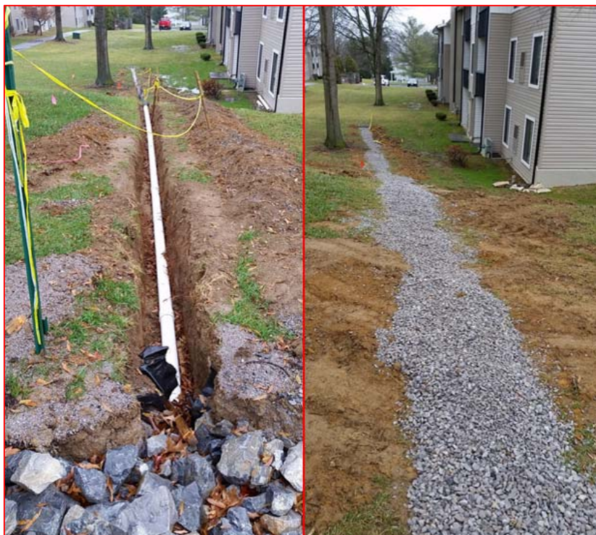
Figure 13. Retrofit of bioretention cell outlet using buried pipe and gravel.
