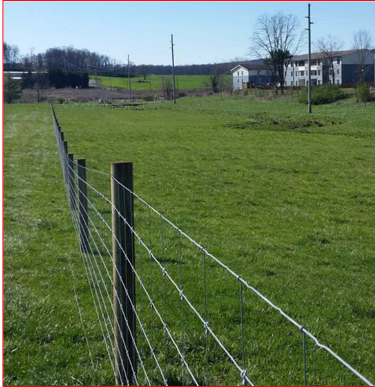
Figure 3. Livestock exclusion fencing along Holtan Branch looking downstream.
