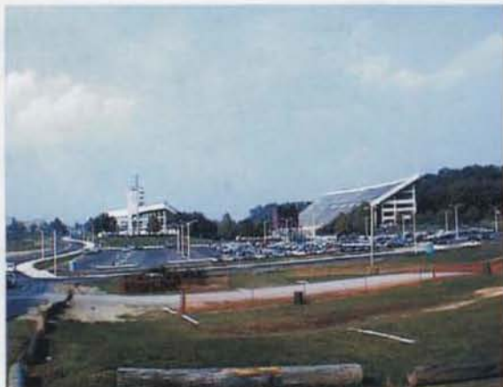
Stadium Parking Lot
