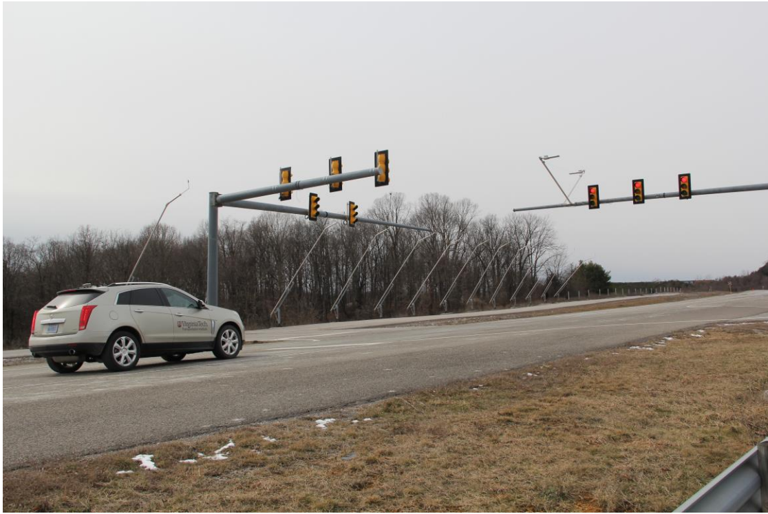
Figure 4-1 Signalized intersection in the VA Smart Road Test facility
