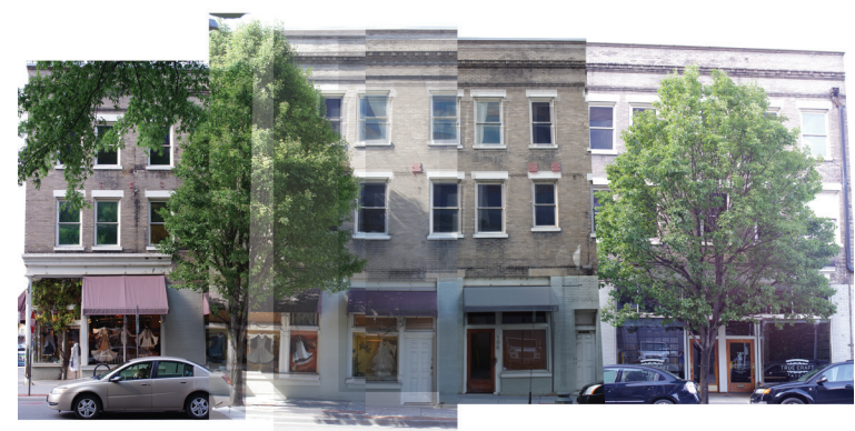
Figure 15 Church Avenue Storefronts
