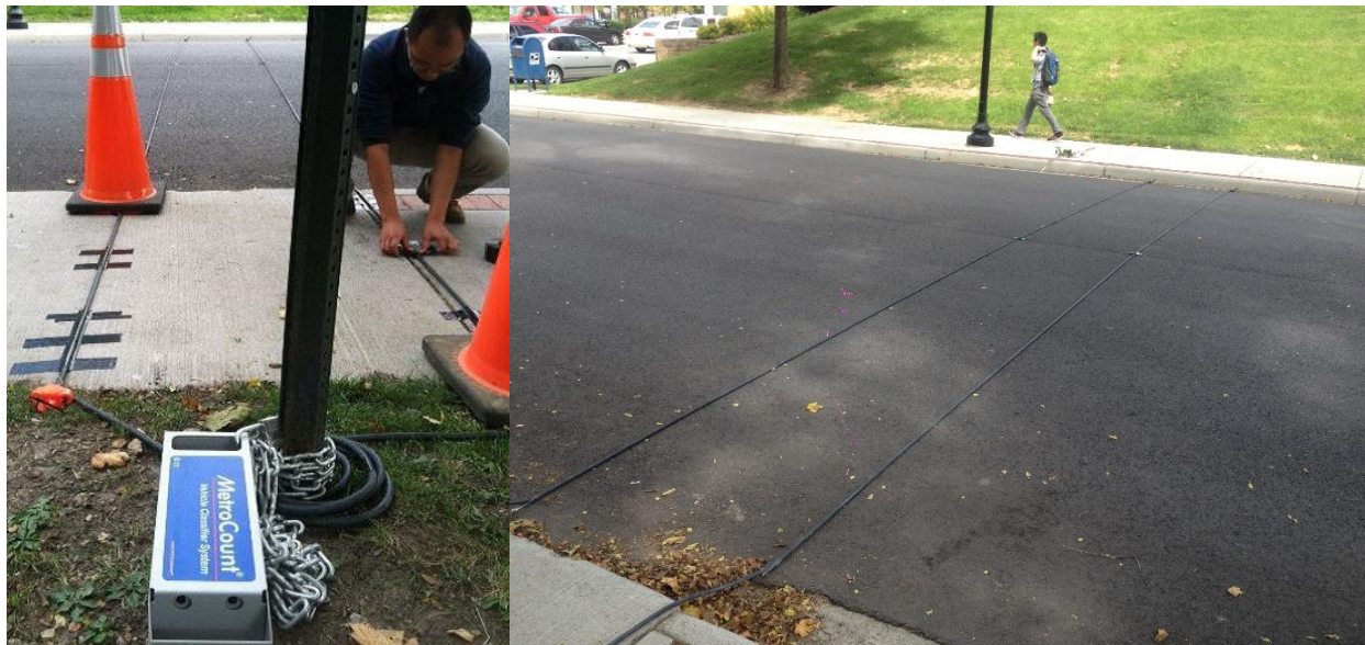
Figure 3. MetroCount counter installation.
