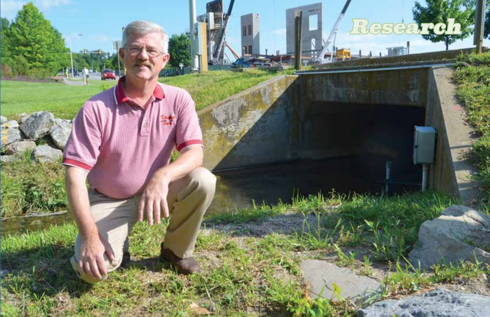
Randy Dymond kneels at a culvert along Stroubles Creek, where a water sensor and related technology can monitor water quality and quantity, and rain levels.
