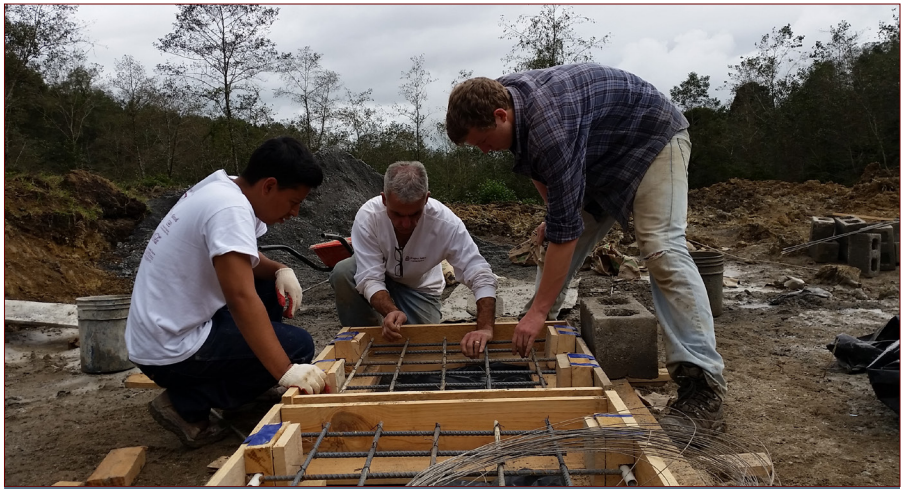
Civil engineering student Marvin Merida, civil engineering alumnus and Engineers Without Borders mentor Rick DiSalvo, and mechanical engineering student Joe Buellesbach work on hatches for a septic tank in Xix, Guatemala.
