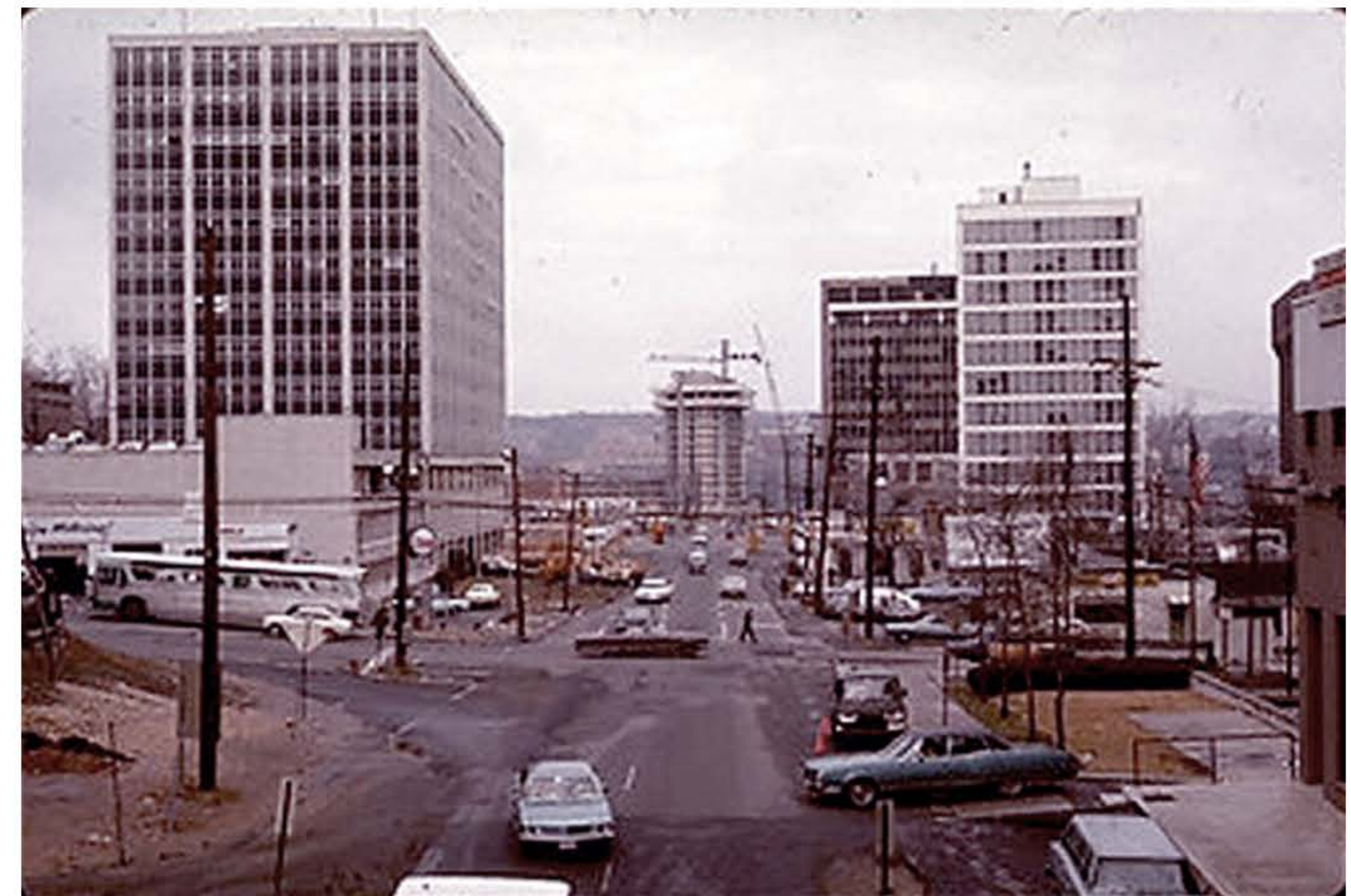
Figure 8. Circa 1960 Looking up N. Fort Myer Drive towards the Key Bridge Marriott 10
