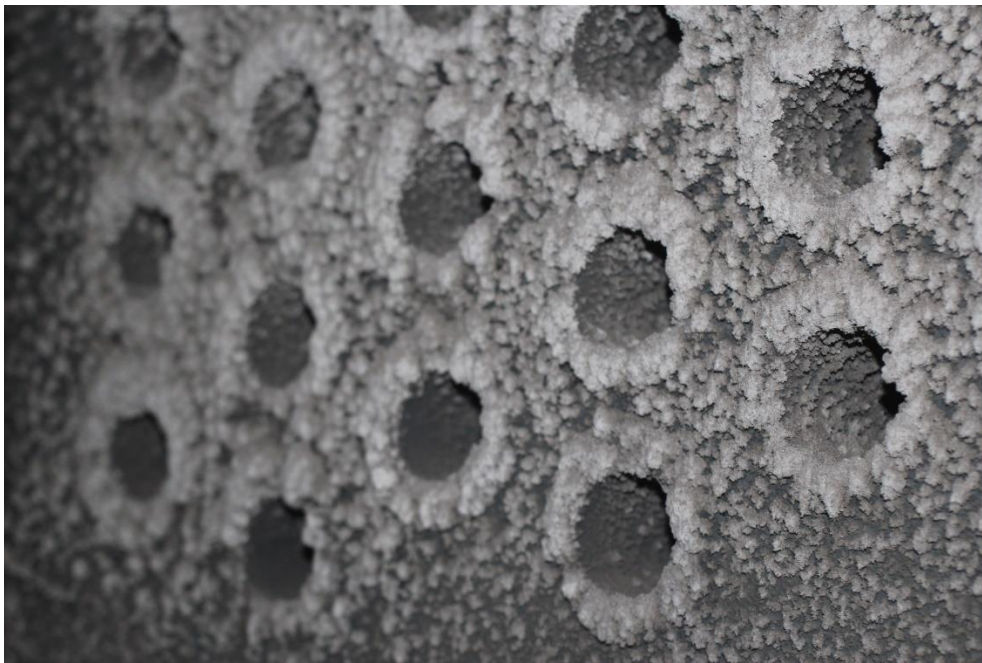
Figure 3.3. Ash build up in the heat exchanger lowers curing efficiencies and increases fuel consumption. The combustion chamber (upper) collects larger pieces of ash in close proximity to the wood pellet burner compared to the secondary tubes (lower) that generally collect the smaller fly ash particles.
