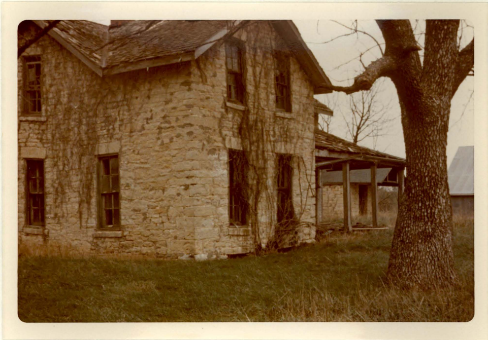
Fig. 81. Stone taken from under the sod close by gives this home its character. Notice the rough surface and large corner stones used. Such homes, barns, as well as the stone fence posts and stone bridges, create the strong regional landscape character of the Smoky Hills "Land of the Post Rock."
