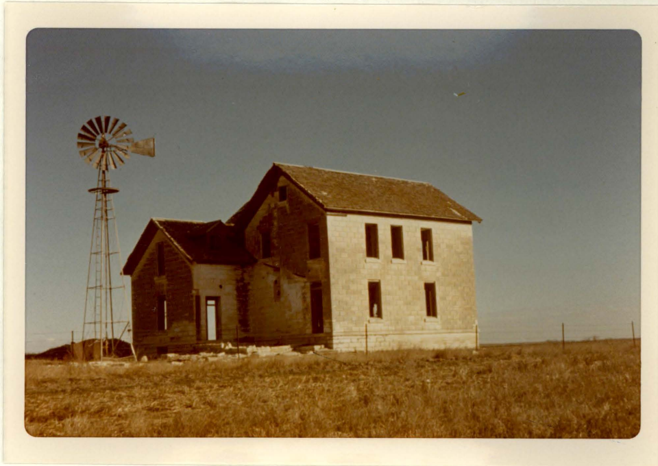
Fig. 83. The roof line still straight, the whole structure even in its dilapidated form, still shows strength. The architectural line was rigid. Native building stone was worked down to a smooth finish. These homes are monuments to a recent past and are bold elements in the wide landscape.
