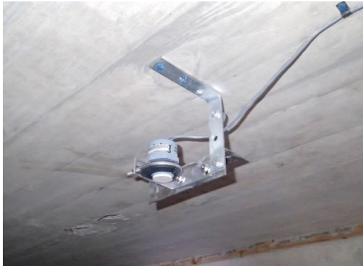
Figure A.1 – The Massa M-300/95 mounted on the soffit of a concrete box culvert
