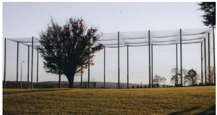
The drone cage was recently developed in September. It is approximately 300 feet long, 180 feet wide, and 80 feet high.
