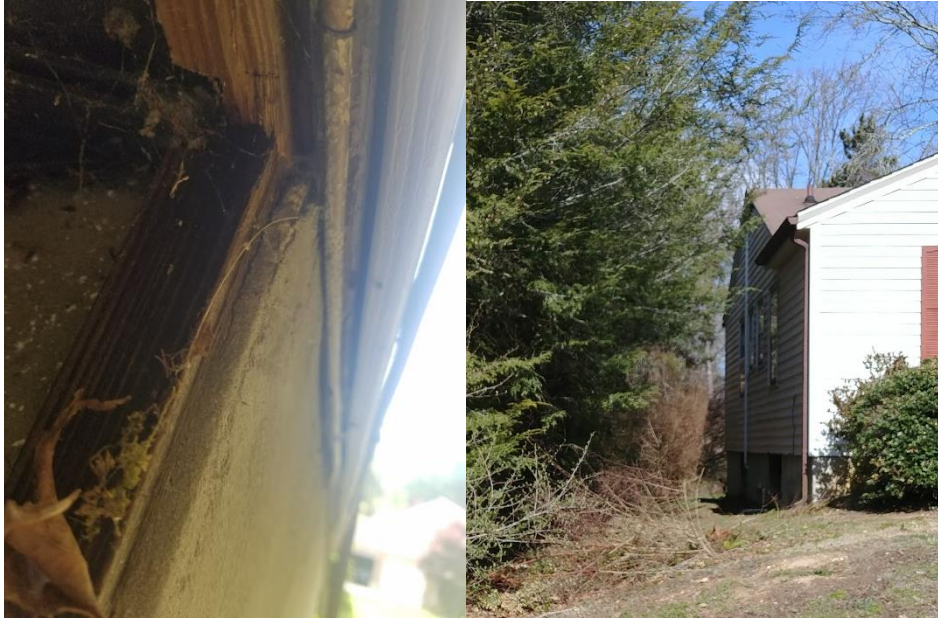
Figure 2.4: (Left) The opening under the cladding at the joint between it and the masonry, at the corner of a basement window. (Right) The high activity side of the house with adjacent trees.
