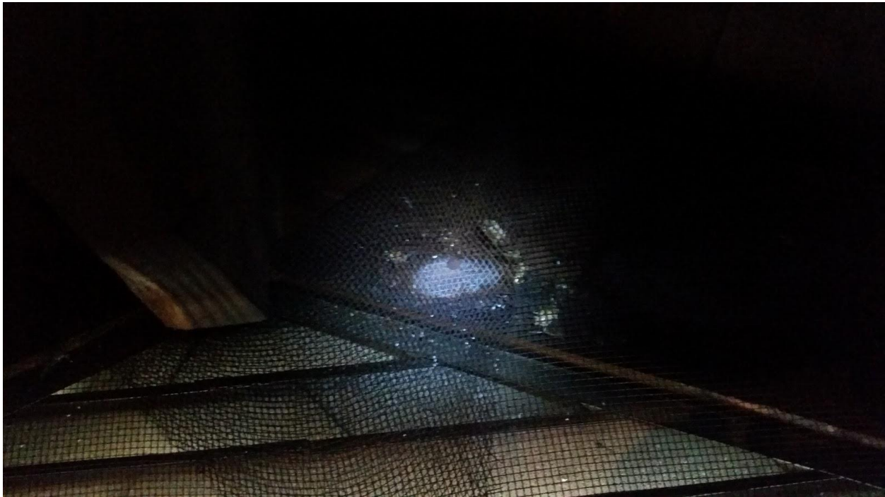
Figure 4.1: Metal screen inside an attic gable vent in Blacksburg, VA, with trapped dead H. halys illuminated by the flash. The vent on the other end of the building had no screen.
