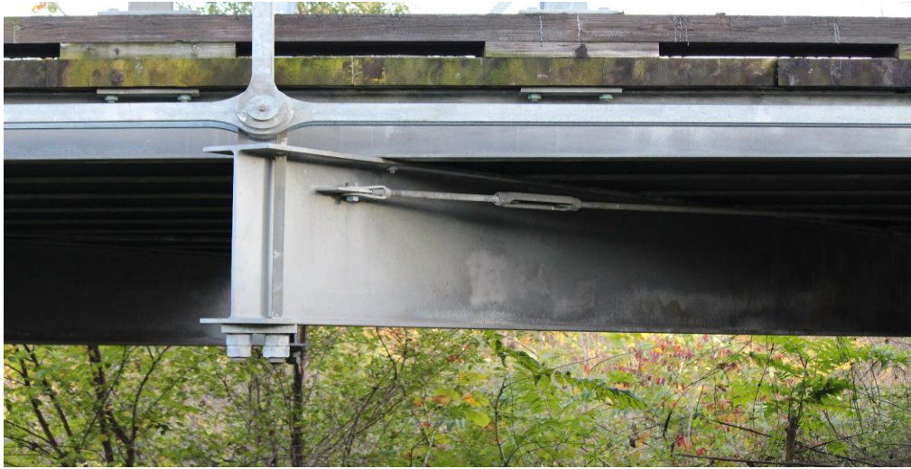
Figure 4: Galvanized Bridge Components (Goshen Land Company Bridge, VA)
