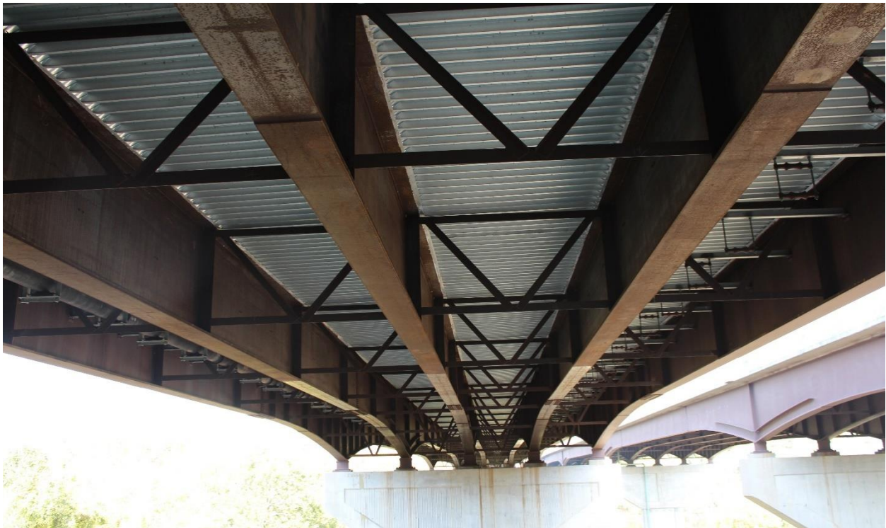
Figure 7: K-Bracing Systems Welded to Gusset Plates (Lee Highway Bridge, Radford)
