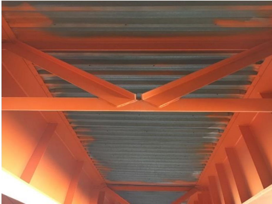
Figure 3: Painted Girders and Bracings in a Bridge (Highway 460, Blacksburg VA)
