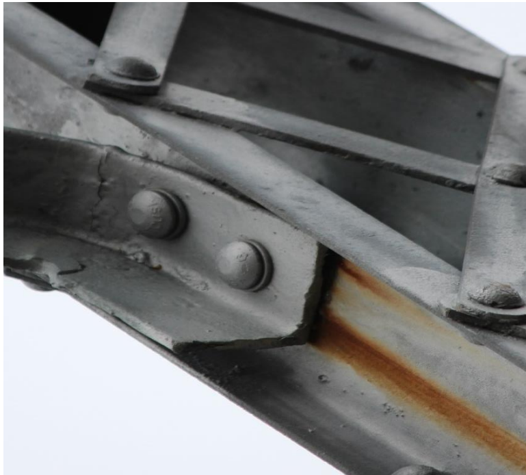
Figure 9: Rust Bleeding (Goshen Land Company Bridge)
