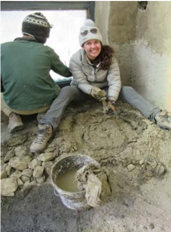
SBIO major Lauren Holt (left) mixing a batch of mud to cover interior walls while Sara Hernandez (Sr. Mech. Eng.) applies the mix to the walls.
