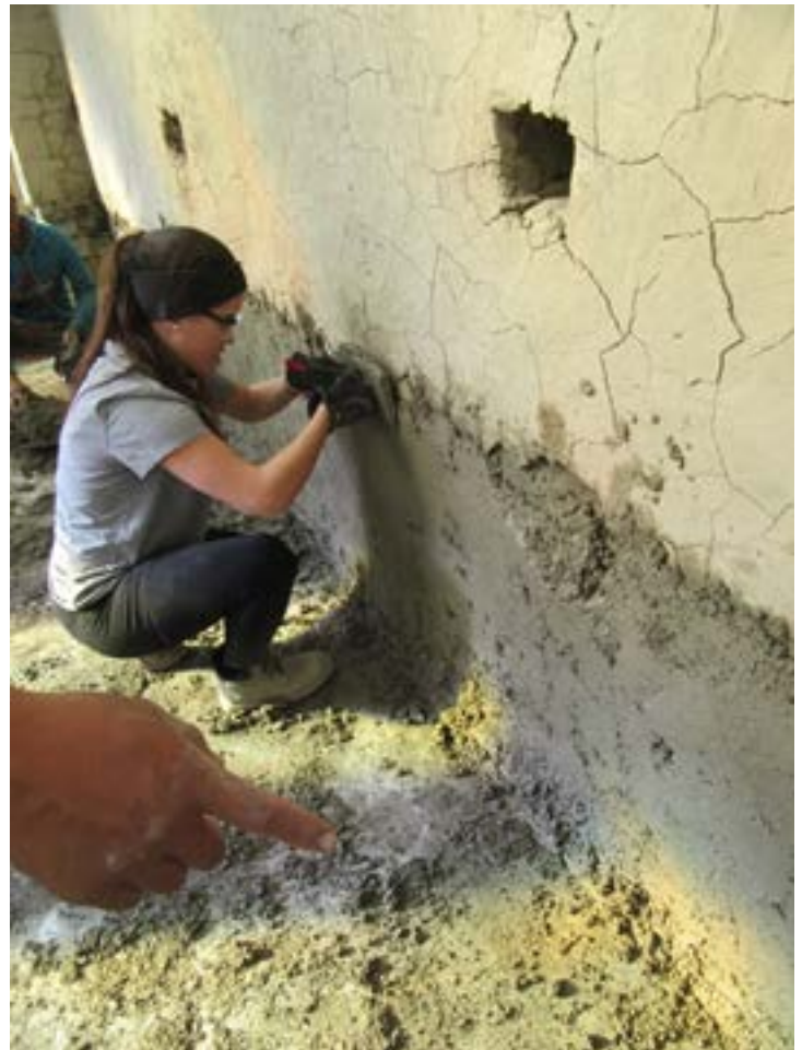
SBIO major Lauren Holt (left) mixing a batch of mud to cover interior walls while Sara Hernandez (Sr. Mech. Eng.) applies the mix to the walls.
