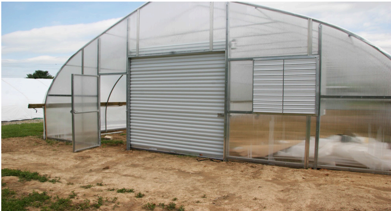
The new high tunnel built at the Urban Horticulture Center in 2014.
