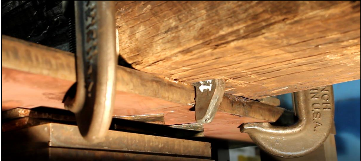
Figure 94: Hook engagement of the Lewis Forged hook bolt with the edge of the steel plate.
