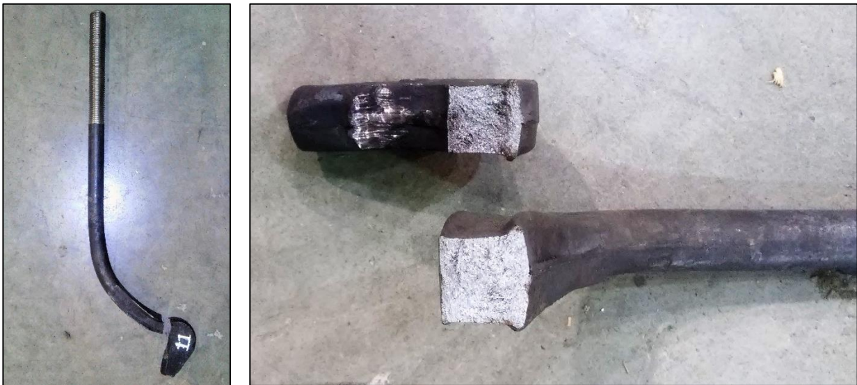
Figure 95: Fracture in Lewis Forged hook bolt – Fastener 11
