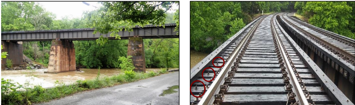
Figure 17: 4784 West River Road - Hook bolts spaced at every 2 nd tie
