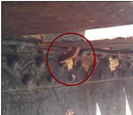
Figure 19: Loose hook bolt from Glade Creek bridge Figure 20: Loose hook bolt from Berkley Road bridge
