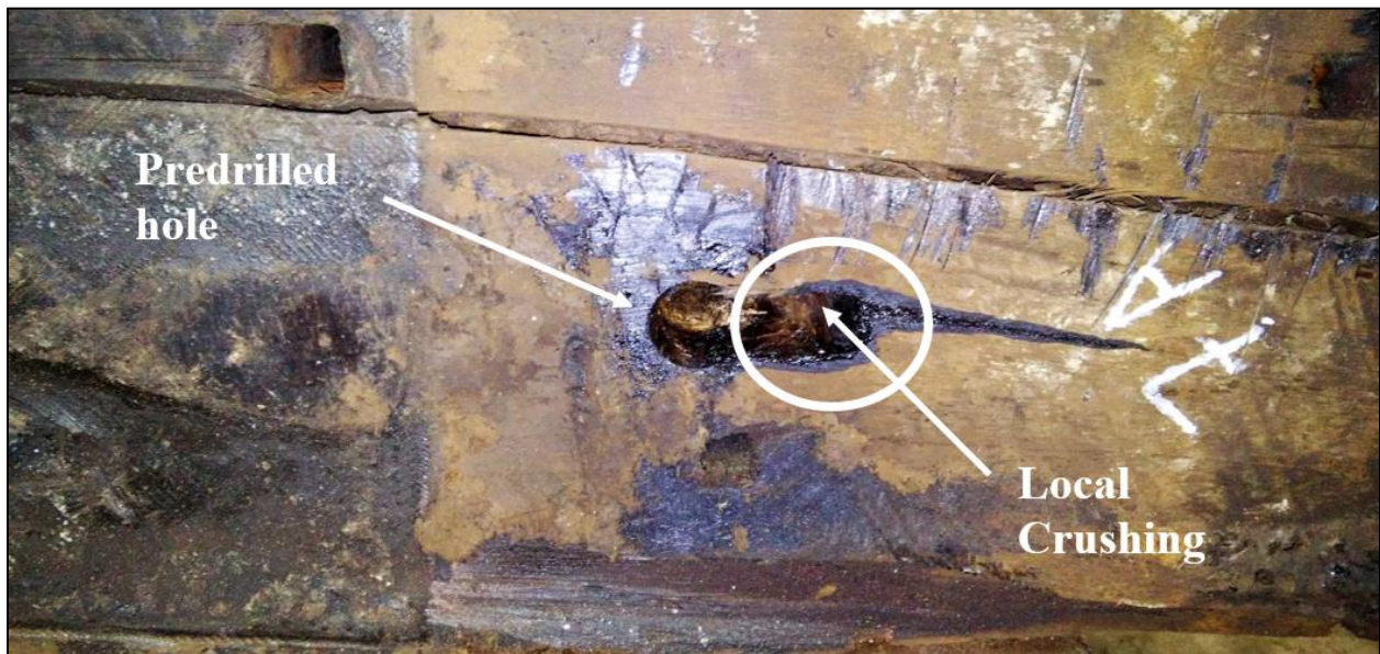
Figure 87: Local crushing of the wood near the fastener
