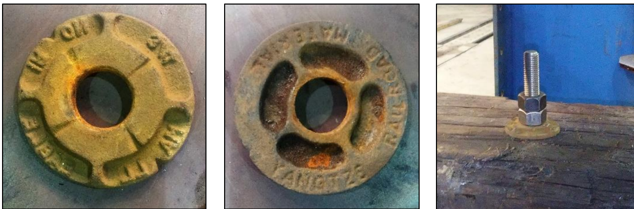
Figure 52: Bridge washer and round body hook bolt secured with two nuts
