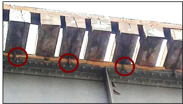
Figure 16: Hook bolts spaced at every 2 nd tie
