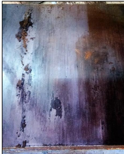
Figure 77: Steel plate after lateral push tests on Tie 6
