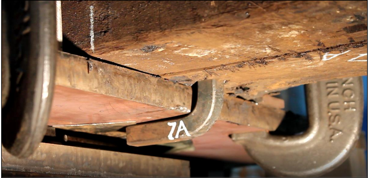
Figure 50: Installed square body hook bolt
