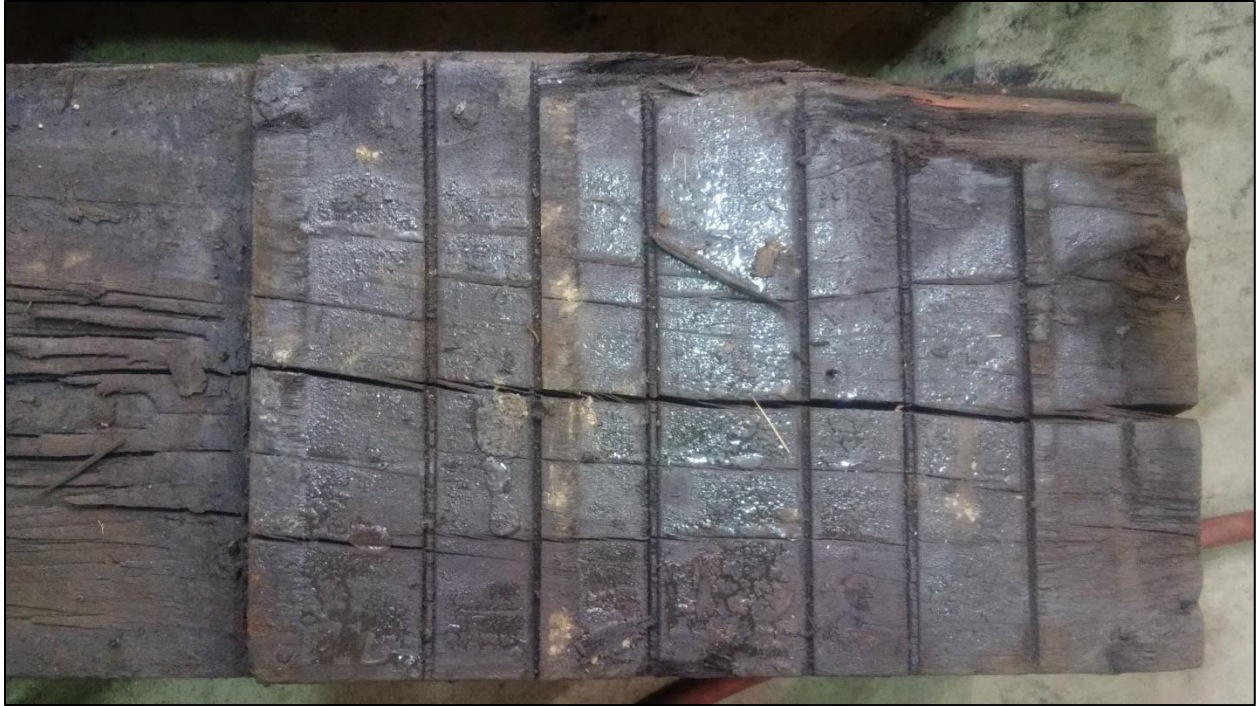
Figure 37: Grease on bridge tie
