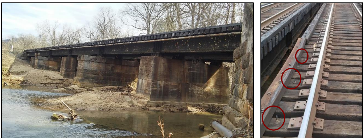
Figure 11: Glade Creek Bridge - Hook bolts at every 3rd tie
