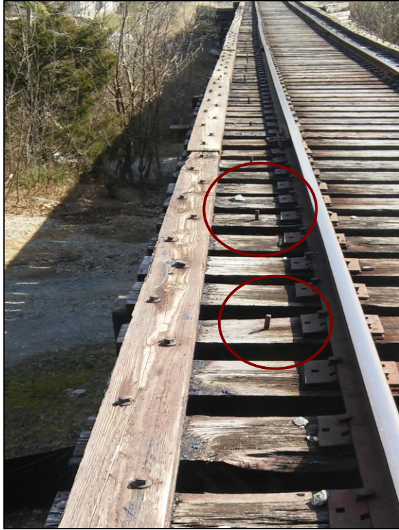
Figure 21: Missing nuts on hook bolts
