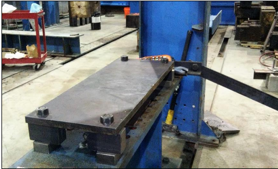
Figure 42: 14" x 30" steel plate attached to the W27x235 bridge girder section
