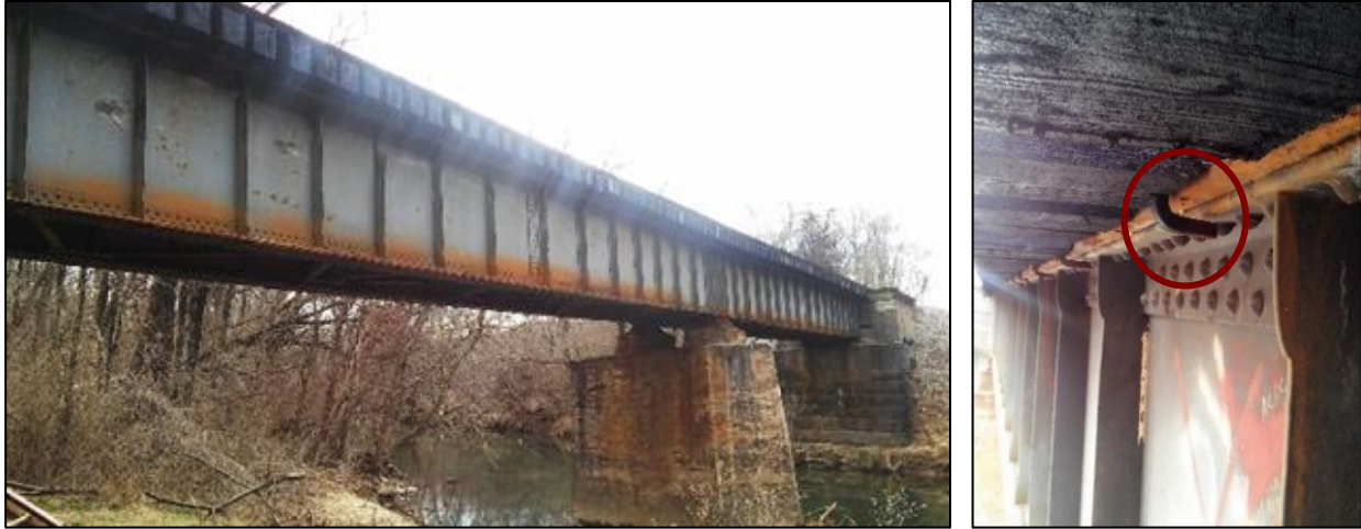
Figure 10: Berkley Road Bridge - Riveted girders with hook bolts
