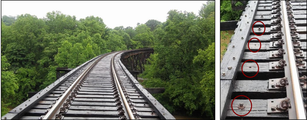
Figure 18: 4829 SW River Rd - Hook bolts spaced at every 2 nd tie
