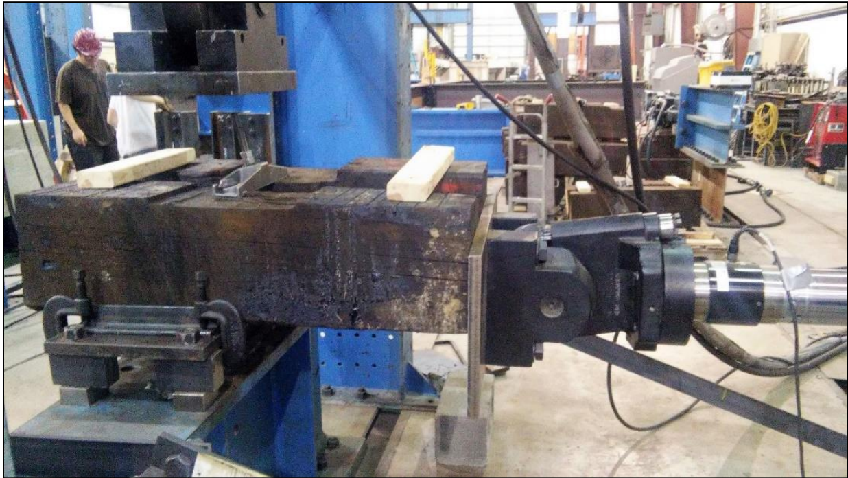
Figure 55: Installation of Quik-set anchors
