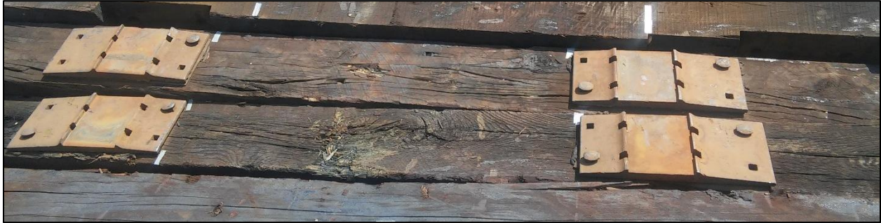
Figure 38: Bridge ties having tie plates, bearing pads, railroad spikes and hook bolts
