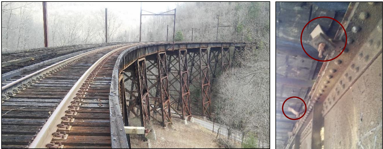
Figure 13: Bridge across Highway 10, WV - Clip anchors at every 4 th tie
