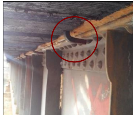
Figure 19: Loose hook bolt from Glade Creek bridge Figure 20: Loose hook bolt from Berkley Road bridge
