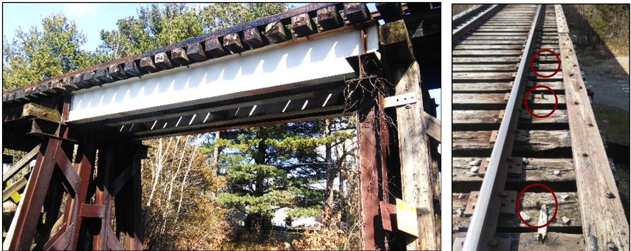
Figure 12: Ellet road bridge - Hook Bolts at every 4th tie
