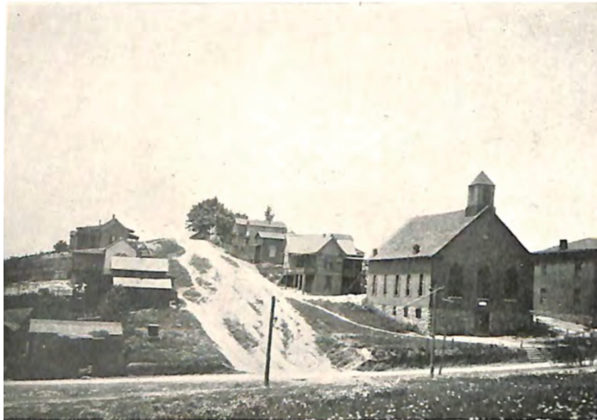
Figure 8. Photo from Nolen's Remodeling Roanoke, 1907, to illustrate the problems in the African American section of town. In particular, Nolen was especially concerned with the grades of the roads that were not only ineffective but unattractive. Nolen wanted to rework the layout of the streets in that section to incorporate the natural landscape of rolling hills.
