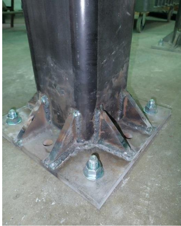
Figure 16: Connection between support beam and ground
