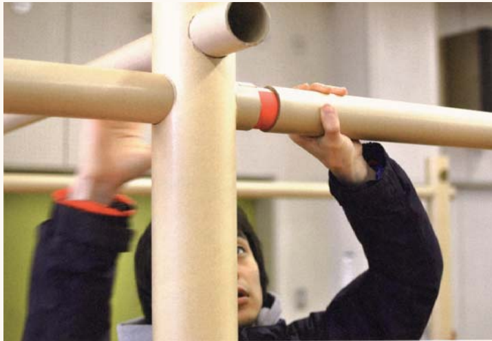
Figure 38. Paper partition system joint [38]
