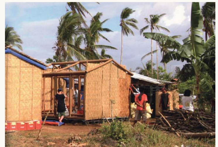
Figure 33. Paper Log House for the Philippines [33]
