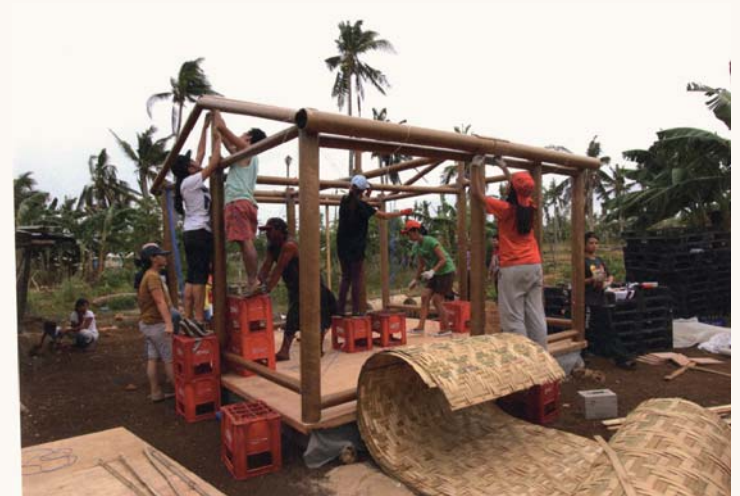
Figure 31. Paper Log House for the Philippines [31]
