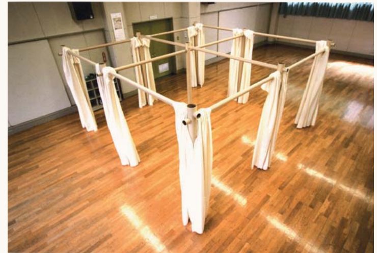
Figure 39. Paper partition system module [39]
