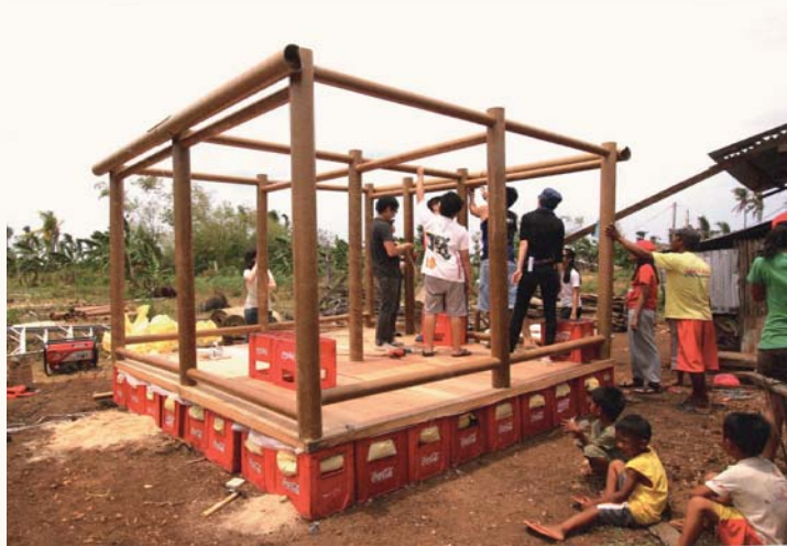
Figure 30. Paper Log House for the Philippines [30]
