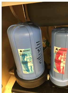
Figure 1-2 The illustration of a carbon filter on the left taking in effluent from a sediment prefilter on the right
