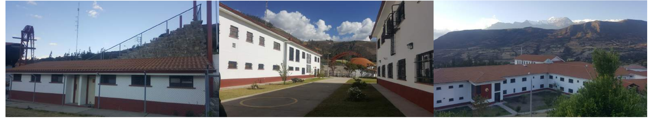
Stone Retaining Wall Amphitheater
