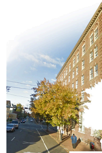
STREET CONDITION AT 601 PRINCE
