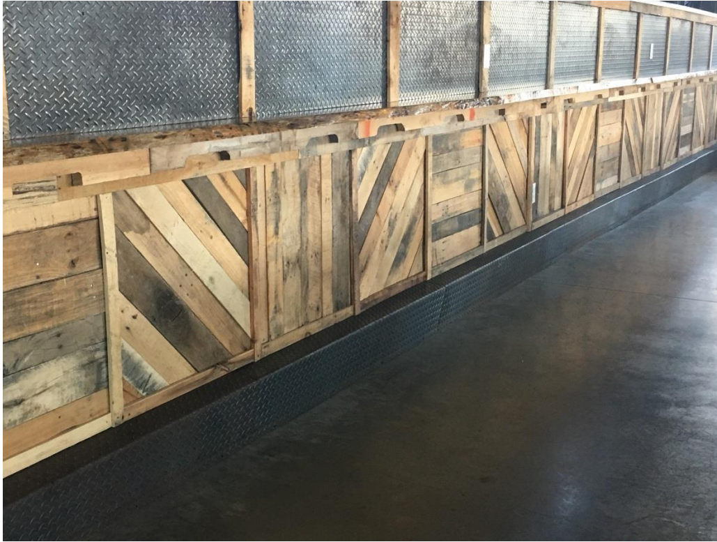
Figure 11 Example of pallet parts being used in new construction at Highland brewery in Asheville, North Carolina.
