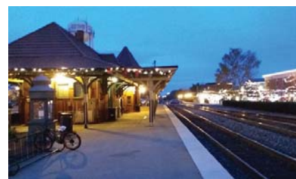
⑧ Old Town VRE Station Situated in Old Town Manassas - a commuter rail station that gives access to the VRE train that goes into Washington, DC as well as a more far reaching, Amtrak train.
