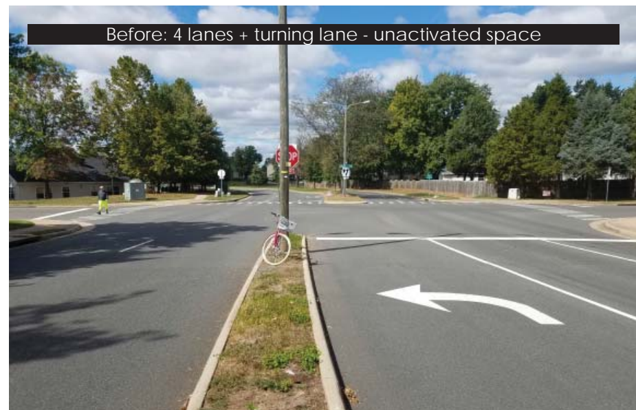
Existing intersection at Cloverhill Road + Hastings Drive
