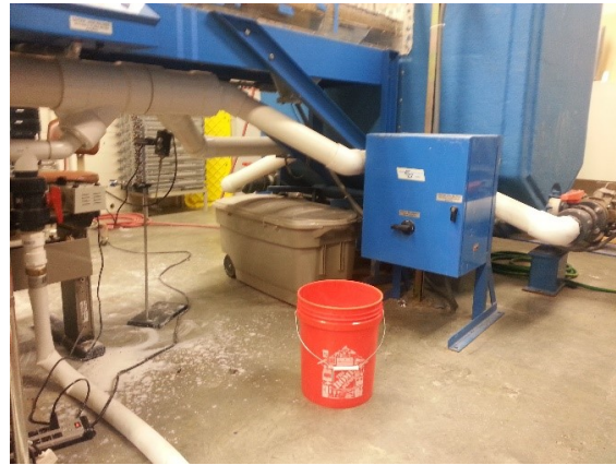
(b) Pump section from flume tank and recirculation piping
