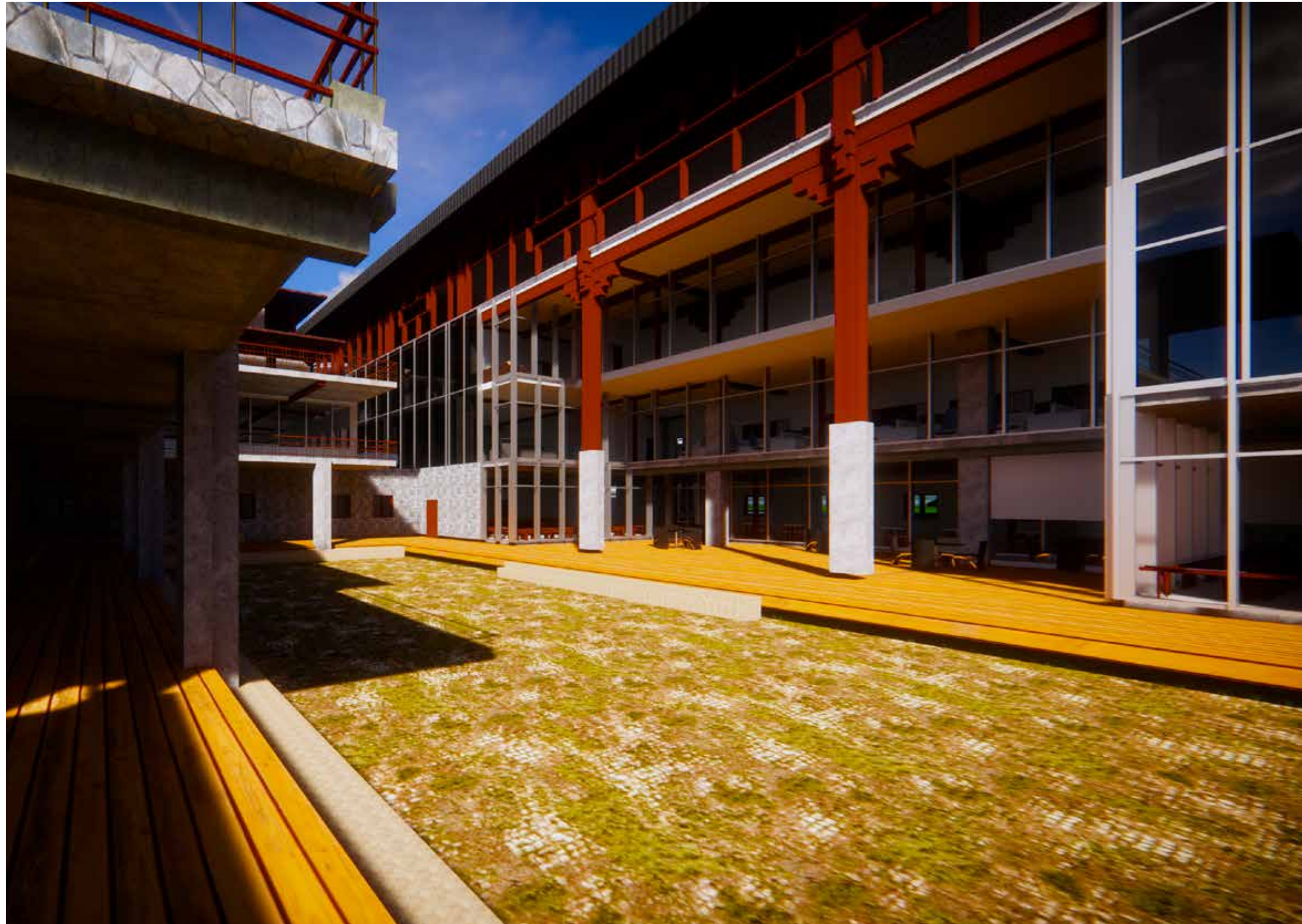
Courtyard view of dougong brackets.
