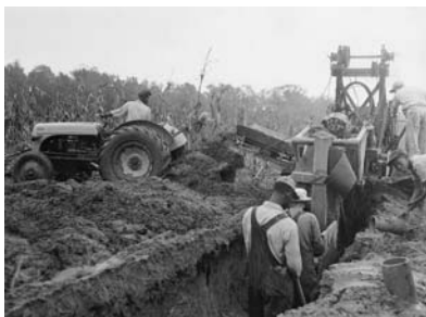
Tile drain installation, late 1910s
