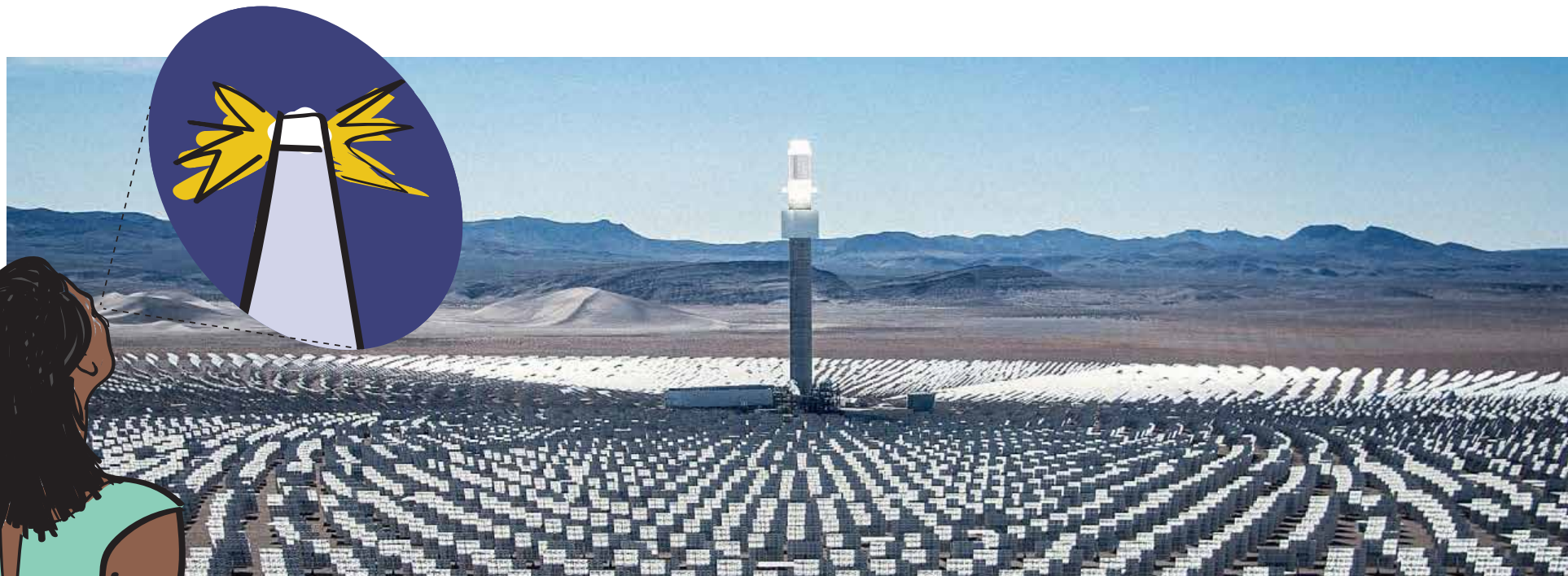
Crescent Dunes Solar Plant - Las Vegas, Nevada
