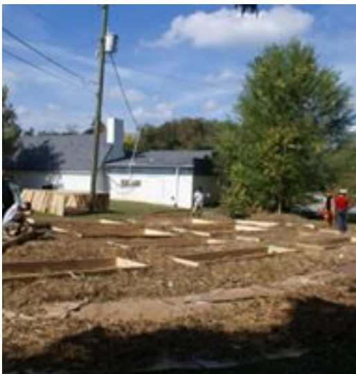
Raised Beds Construction
