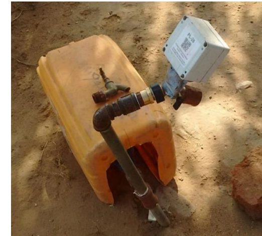
Pressure loggers were installed in one-week rotations at household taps; plus 6-7 weeks at network sampling points.
