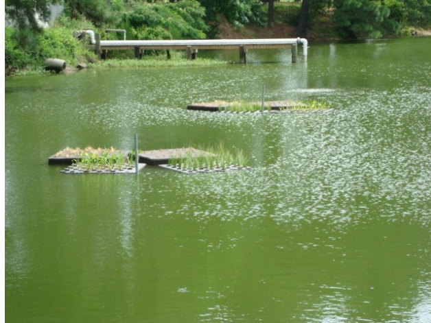
Figure 1.2. Newly planted and installed FTWs (image courtesy of Laurie Fox, Virginia Tech).
