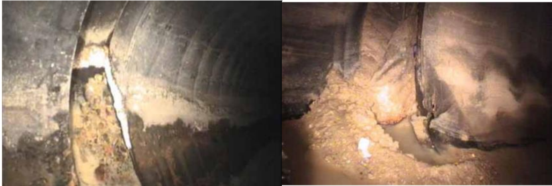
Figure 11: Joint Displacements. Source: Abolmali, A., Motahari, A. and Hutcheson J.(2010)
