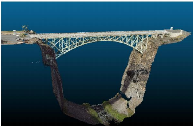
Figure 2.2.1 - 3D Point Cloud of Crooked River Bridge (Gillins et al., 2018)
