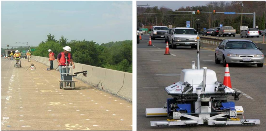
Figure 2.4.4 - Automatic Robotic Crack Detection (Prasanna et al., 2016)
