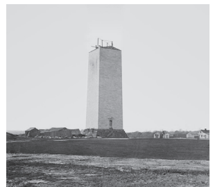
Uncompleted Washington Monument in 1860
