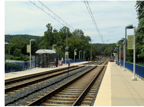
Figure 6.16: Warren Road Station
