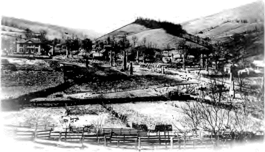
Newport, Virginia, on April 1, 1902, the day after the fire.
