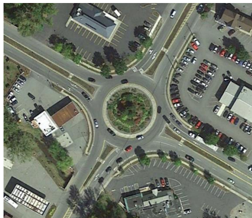
Figure 3-4. A two-lane roundabout in Brattleboro, Vermont (Google Earth image, accessed August 2016).
