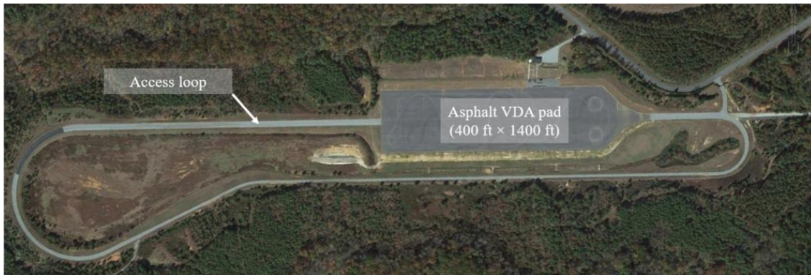
Figure 7-18. Google Earth view of Track 8 area at MLPG (Google Earth image, accessed January 2017).
