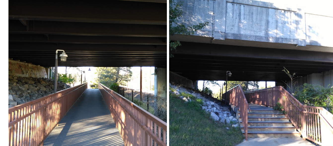
● Connection under the bridge, across the street
